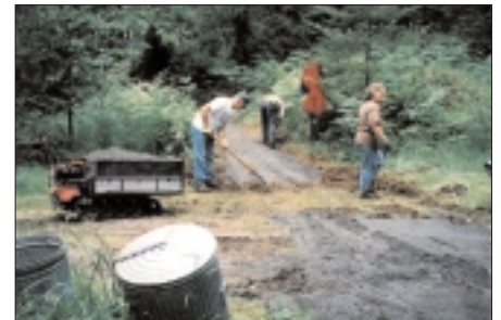
NTD work party hard at work on the Cold Creek Trail.
